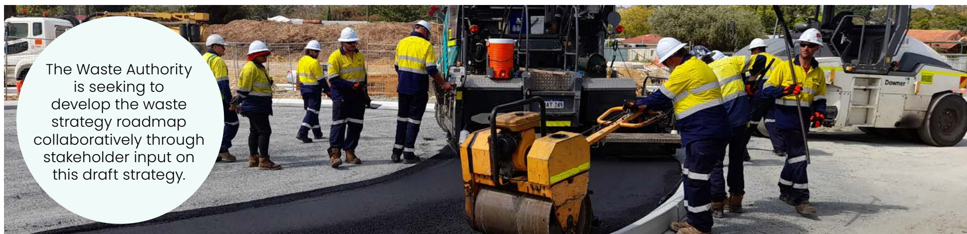
METRONET has used Reconophalt™ – a road surfacing material with recycled content – in its Denny Avenue Level Crossing Removal Project
